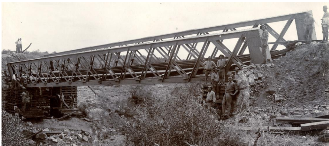
Damaged Metsemaswaane River bridge. National Archives of Botswana
